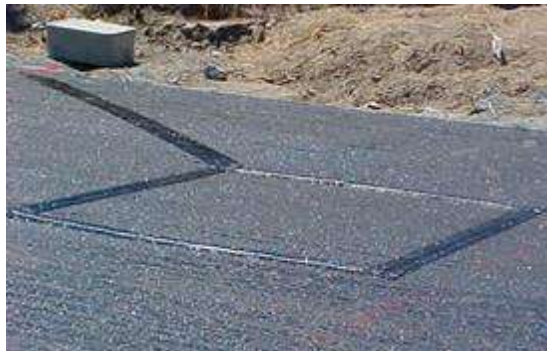
Figure 4-5: Simple loop detector.
